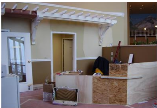
The new reception area undergoing transformation
